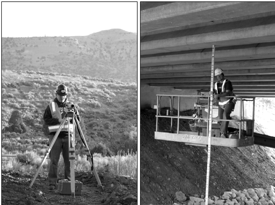
Figure 19. Surveying team for truck load test
