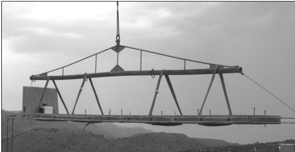
Figure 9. Panel P2-05 being lifted using straps at the bridge site
