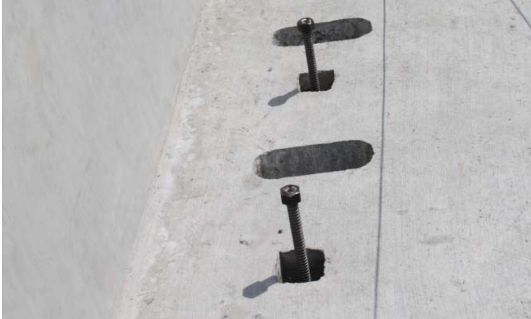
Figure 6. Leveling bolts and shear stud blockouts.
