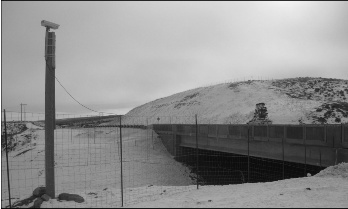
Figure 22. Location of camera with respect to bridge
