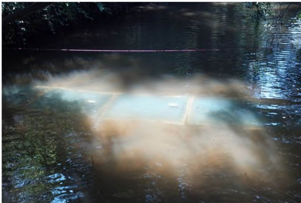
Figure 2.5. Photo of blankets installed lengthwise along a transect at West Bear Creek. Note the near complete coverage of the stream bottom across the transect by the blankets.
