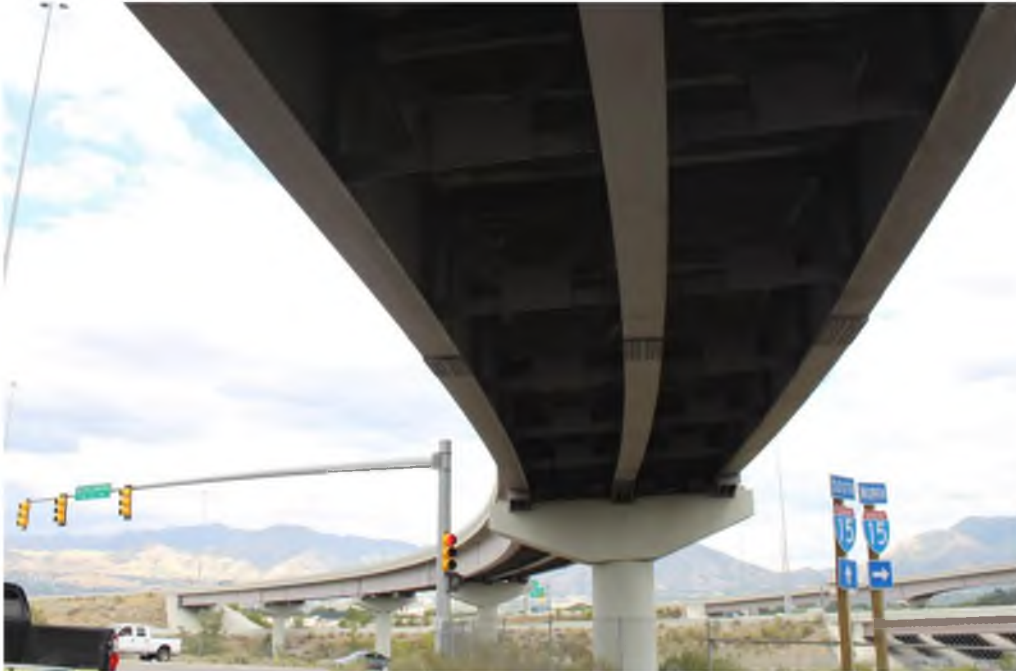
Figure A.7 Site photograph of the curved bridge (Bents 11,12,13, and 14)
