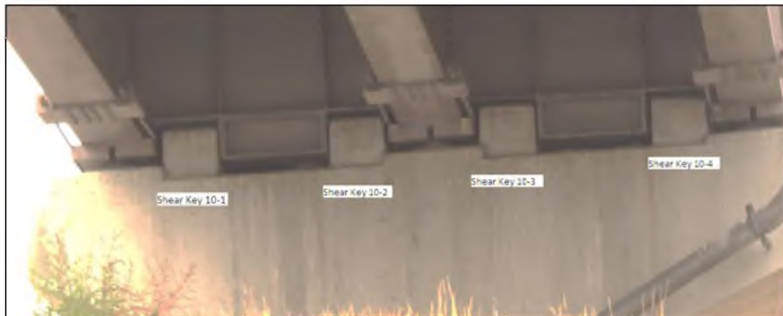
Figure 4.18 Shear keys on the bridge bent
