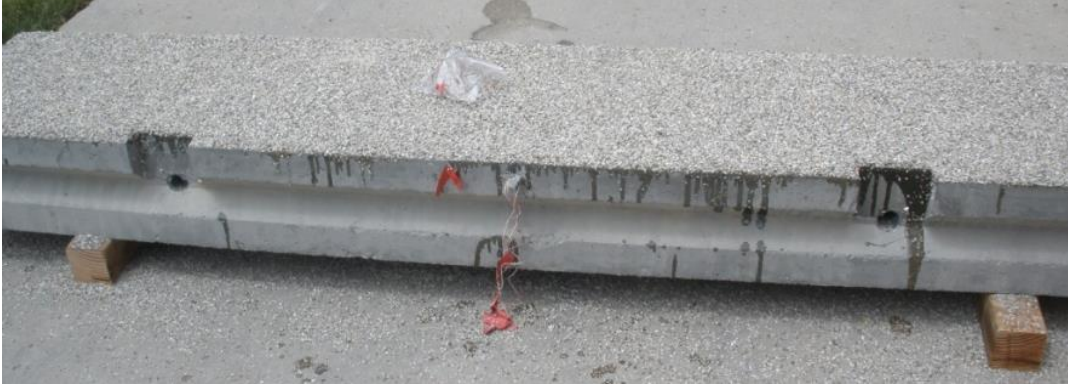
Figure 4.2: Single Panel for Type II Specimen Prior to Grouting;
