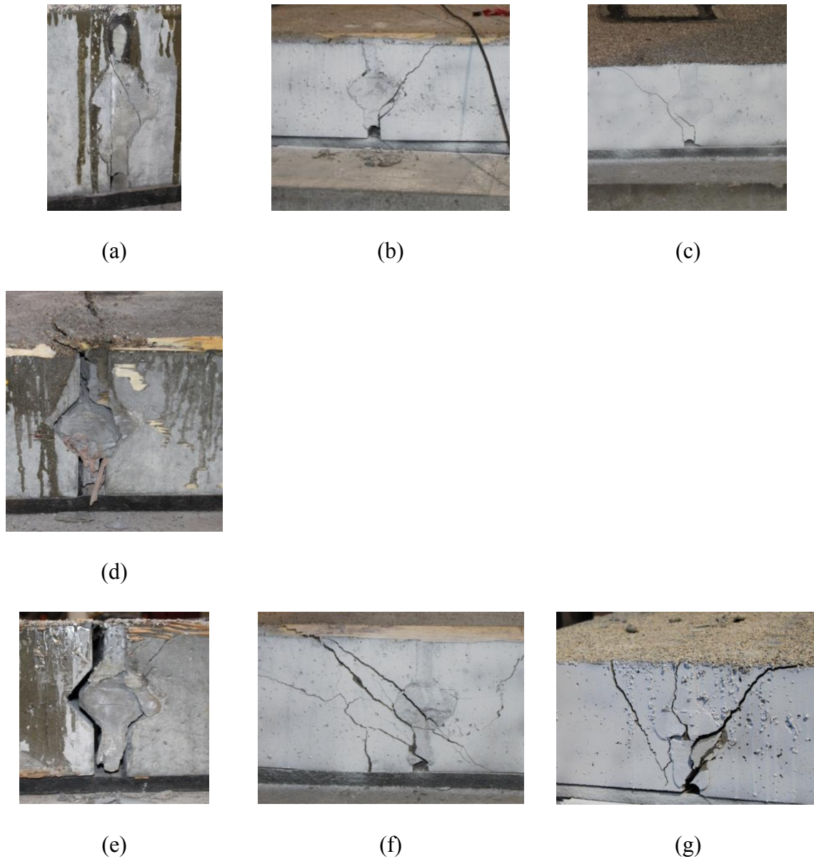
Figure 5.3: Cracking Behavior of the Joint of the Composite Specimens: (a) Initial Crack of Non-Posttensioned Specimen, (b) Initial Crack of 35 psi Posttensioned Specimen, (c) Initial Crack of 48 psi Posttensioned Specimen, (d) Second Crack of Non-Posttensioned Specimen, (e) Joint Cracks after Ultimate Load for Non-Posttensioned Specimen, (f) Joint Cracks after Ultimate Load of 35 psi Posttensioned Specimen, (g) Joint Cracks after Ultimate Load of 48 psi Posttensioned Specimen
