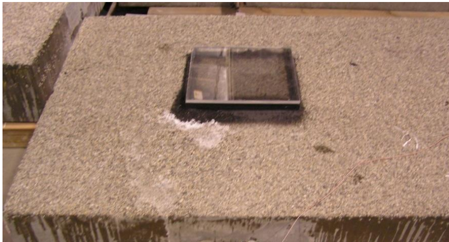
Figure 4.9: Ponding Test Over Grouted Pocket After Cyclic Loading
