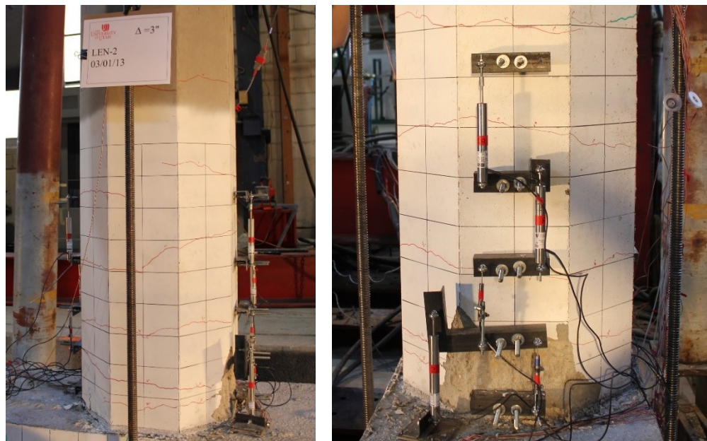
Damage state at 3% drift ratio: cracks and spalling
