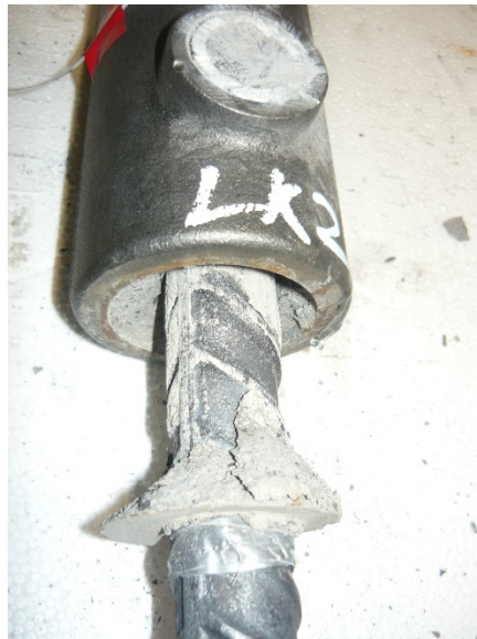
Grout cone failure and reinforcing bar pullout
