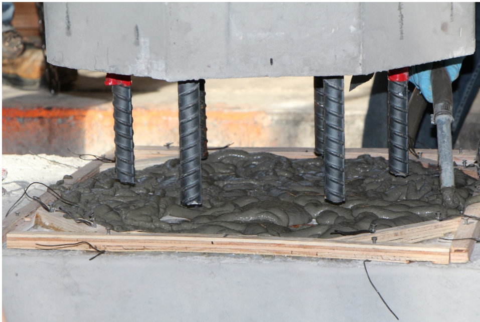
Bed grout at column-to-cap beam interface
