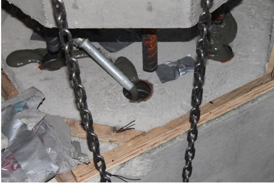
Pregrout technique prior to installation
