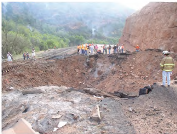
Figure 1. A 24-meter-wide crater produced from an unexpected Deflagration-to-Detonation Transition (DDT) of 16,000 kilograms of high explosives, carried by a truck through Spanish Fork Canyon, Utah.
