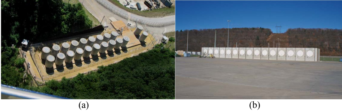
Figure 1.1. ISFSI facilities. (a) Freestanding vertical DSCs on a concrete pad, (b) Horizontal DSC in a concrete vault [4] (This item appears courtesy of IASMiRT at iasmirt.org .)
