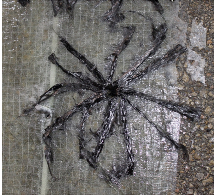
Figure 4.17 – Anchor step 3: Insert into drilled hole and splay the saturated strips.
