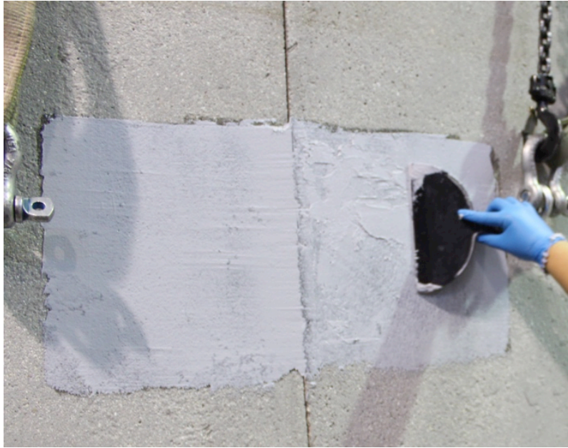
Figure 5.9 – Step 2: Apply epoxy-putty adhesive to primed surface.
