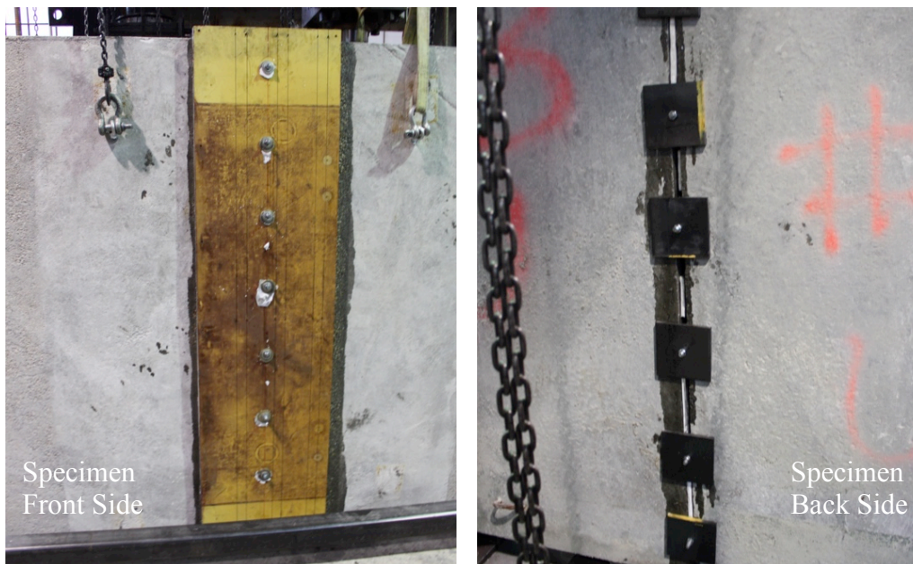
Figure 4.14 – Laminate step 3: Apply pressure with formply, EPS, and all-thread connectors through the seam.
