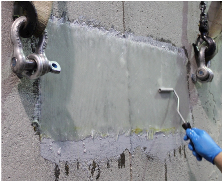
Figure 5.10 – Step 3: Lay-up wet GFRP laminas.
