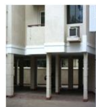
Fig. 1.1: Typical example of OGS building
