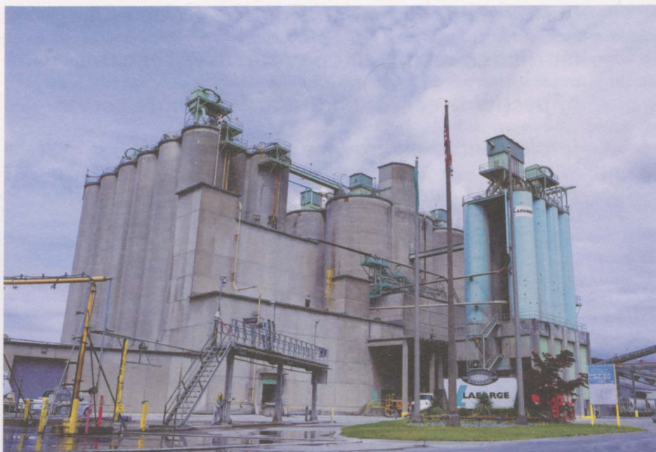
LEFT: Cement companies such as this one in Seattle are some of the largest sources of industrial carbon emissions, according to the U.S. Environmental Protection Agency.
