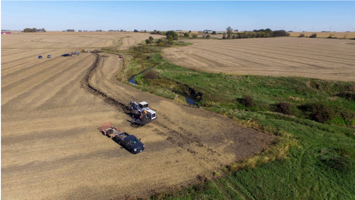
Installation of a saturated buffer in Story County, Iowa. Photograph by Lynn Betts, courtesy of the USDA NRCS and SWCS.
