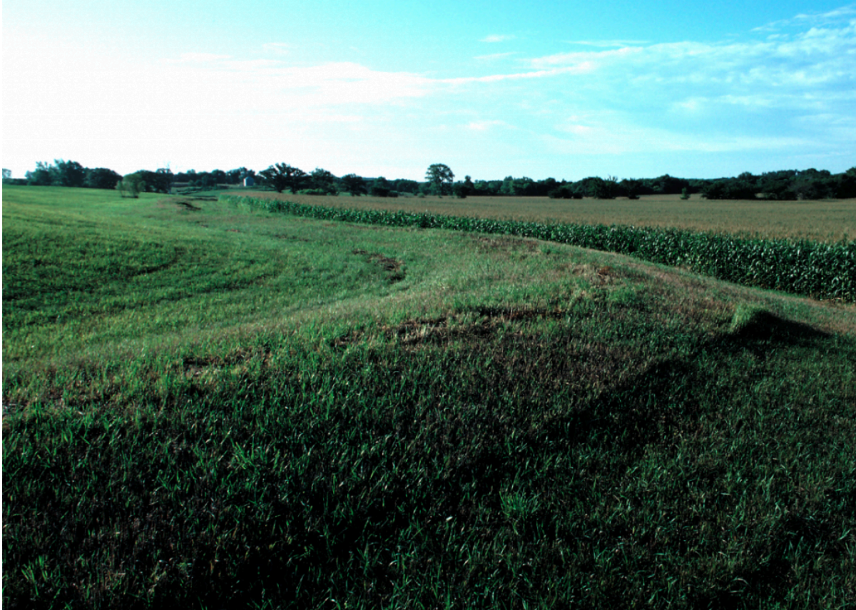
A broad-based terrace forming the down slope ridge for a diversion channel directing water away from the cornfield below. Photo by Lynn Betts, courtesy of the NRCS.
