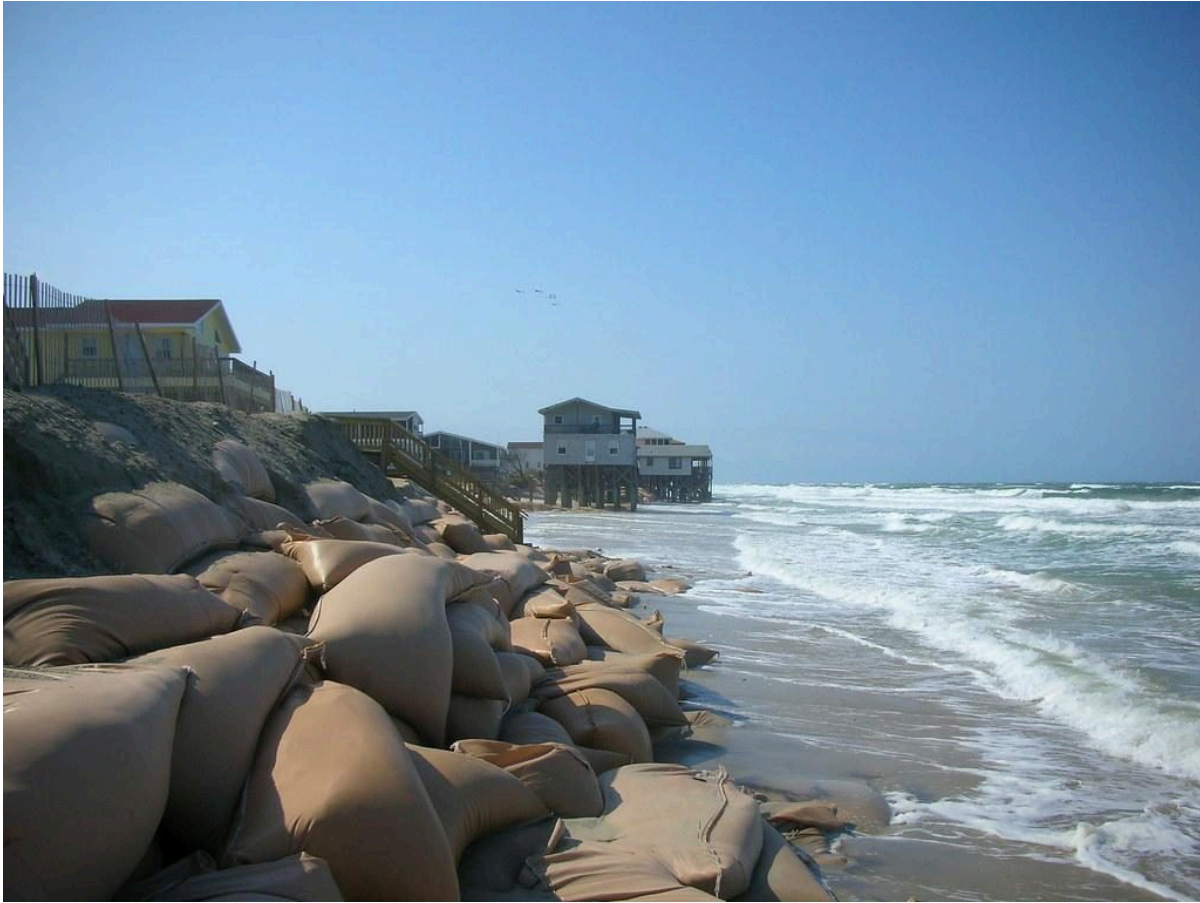
Beach erosion at the Outer Banks of North Carolina. Photograph by David Crouse, courtesy of SoilScience.info.
