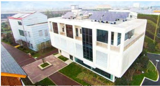
Figure 2 The test building
