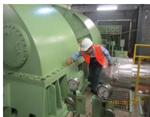
Gambar 17. Memeriksa Instalasi Steam Turbine
