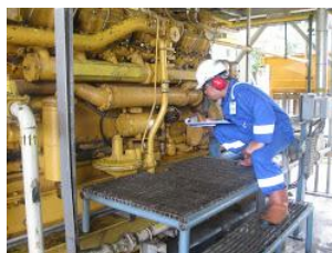
Gambar 13. Memeriksa Instalasi Gas Engine
