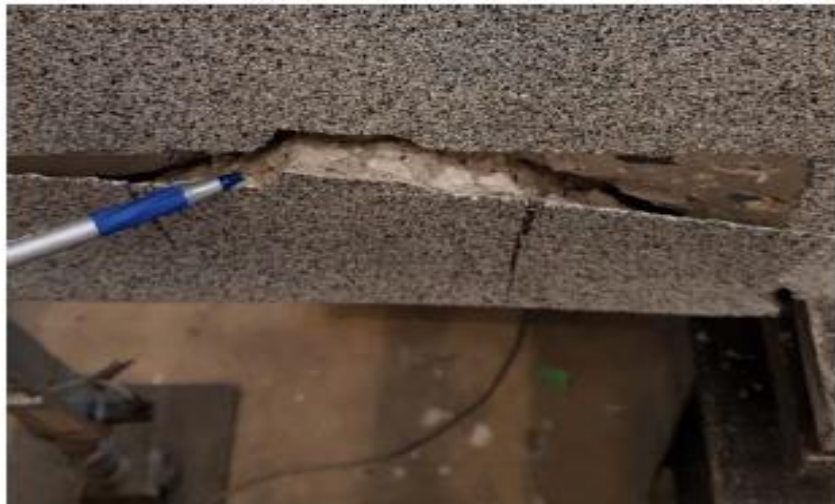
Figure 5.18: Shear-tension failure of strengthened beam (Hughes, 2018)
