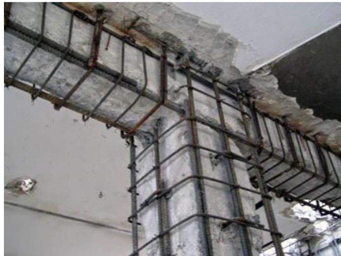
Figure 1.2: Steel Jacketing of columns and beams (Indiamart, 2019)
