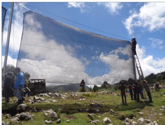
Fig. 2. Repairing an LFC by the community in 2015
