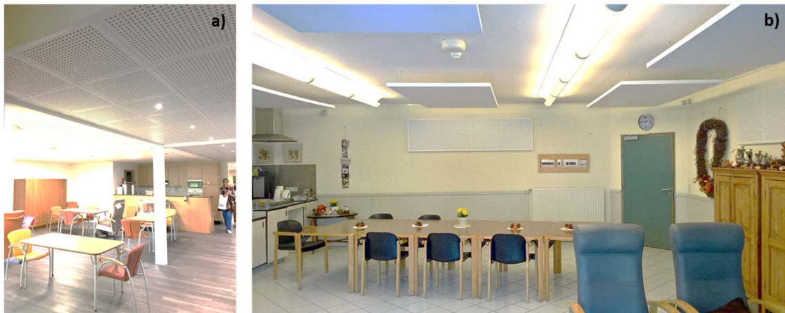
Figure 6 – Overview of the acoustic interventions in the living rooms: a) dining room with absorbing ceiling panels (Gyproc) and acoustic floating floor in VH; b) living room with absorbing ceiling panels (DOX-Acoustics) and wall panels (Gyproc) in LH.
