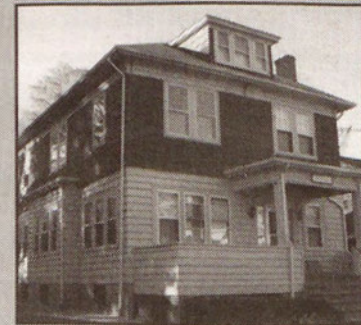
Tollamore 138-140 Radcliffe Avenue
