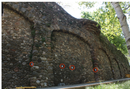
Figure 25. Markers placed on the wall for scaling and calibration
