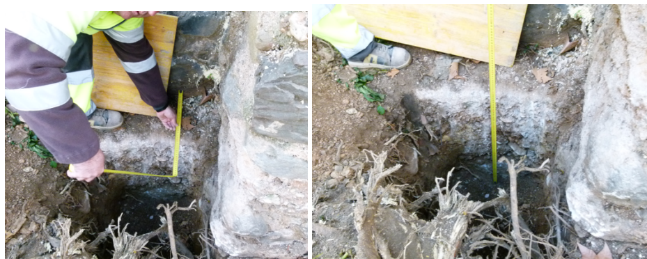
Figure A. 10. Concrete base found in Pit 12
