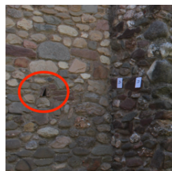
Figure 43. Drainage holes that enabled measuring the wall thickness
