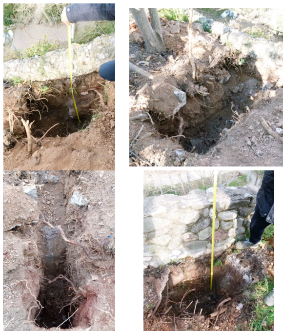
Figure A. 18. Pit 17 on the key of Arch 9 from different angles
