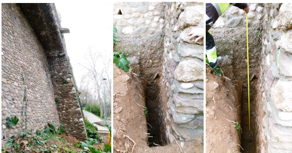
Figure A. 20. Pit 18 on Buttress 9-10
