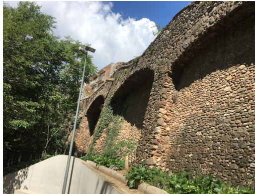
Figure 20. Arches 8 and 9 of Mur Casa Salvans
