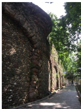
Figure 19. The cantilever balcony section between Arches 6 and 5
