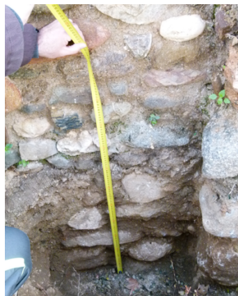
Figure A.2.Pit 3 below Arch 3, on the left side of Buttress 2-3
