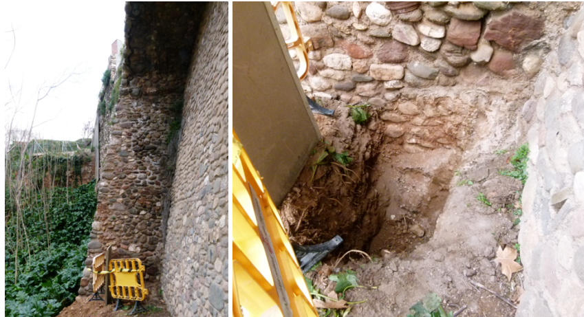
Figure A. 22. Pit 21 on Buttress 10-11
