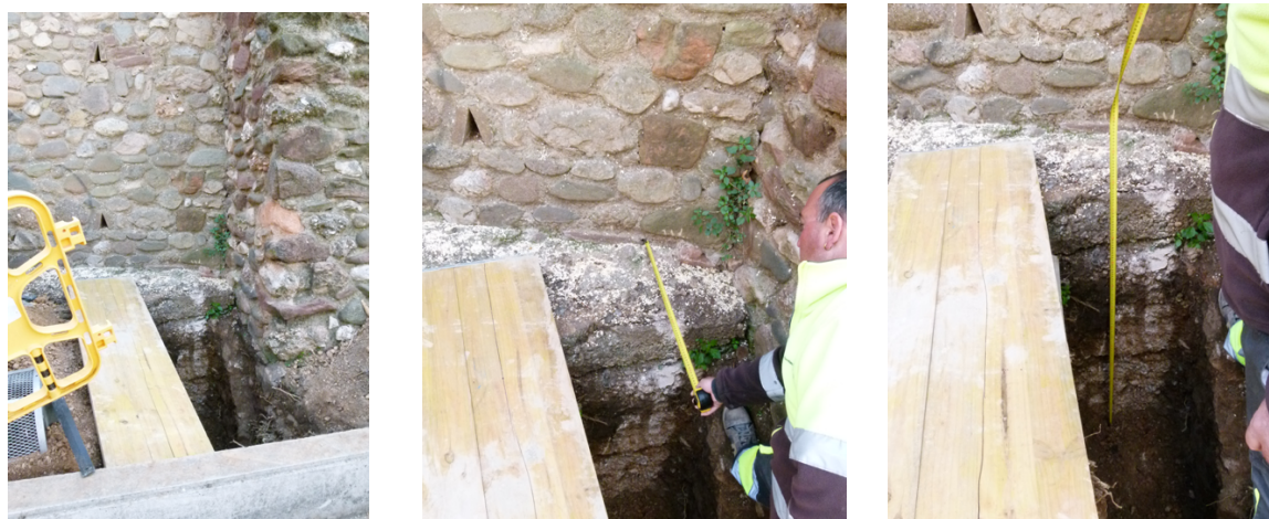
Figure A. 15. Concrete base found in Pit 15
