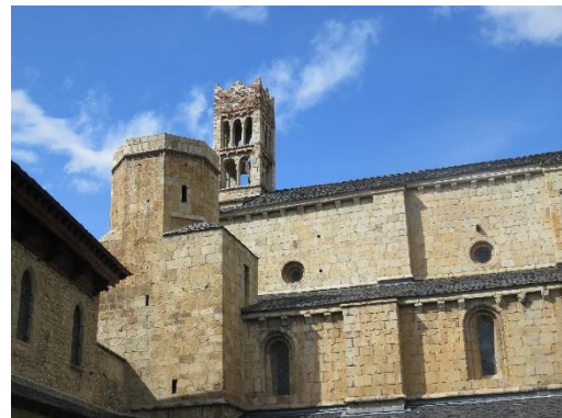
External view from the cloister
