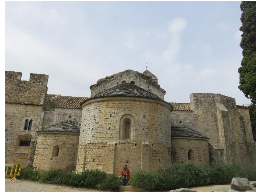
External view of the apse
