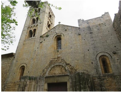
Figure 3.20. Main façade of Santa Maria de Vilabertran
