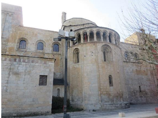
External view of the apse
