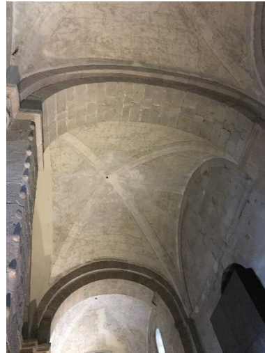
Vault of the aisle
