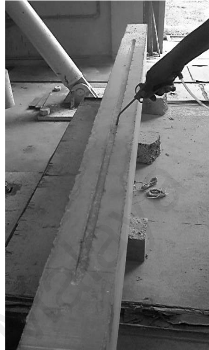
(b) Removing dirt from groove by air jet
