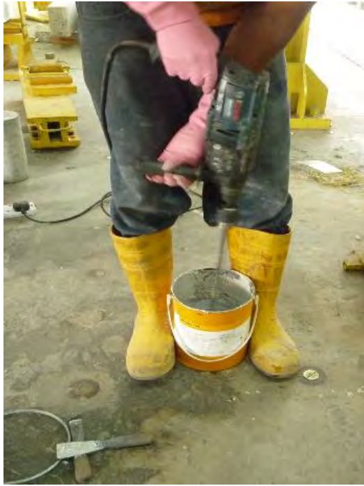
(d) Mixing of two-part epoxy
