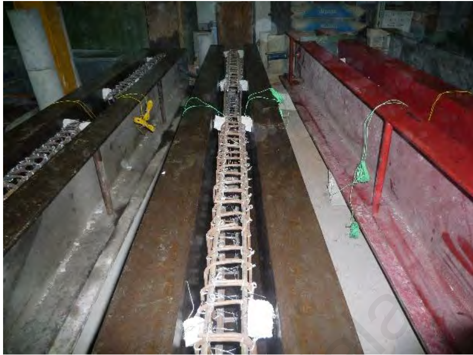
(c) Prepared steel mold for casting
