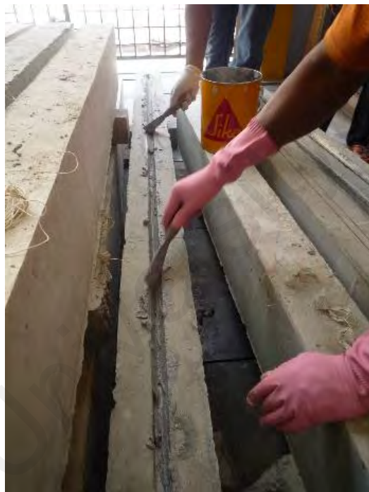
(f) Application of epoxy in groove
