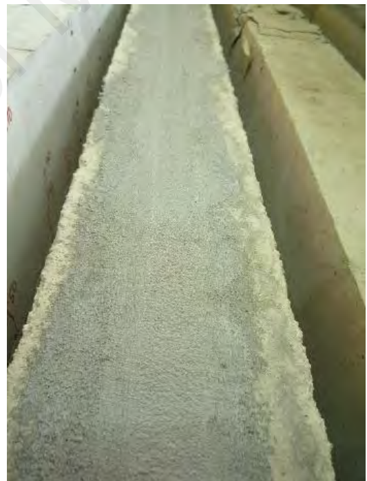
(g) Finishing of the beam soffit
