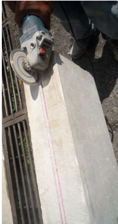
(a) Cutting groove with diamond cutter blade
