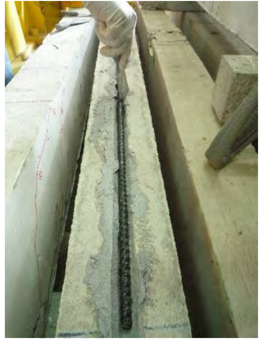
(e) Pressing strengthening bar in epoxy
