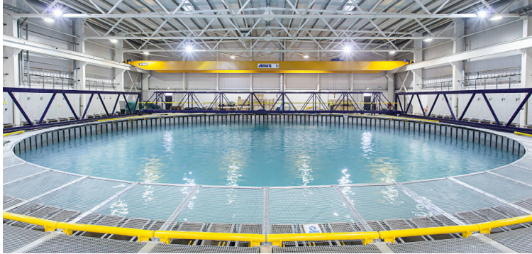
Figure 3: The FloWave Ocean Energy Research Facility.
