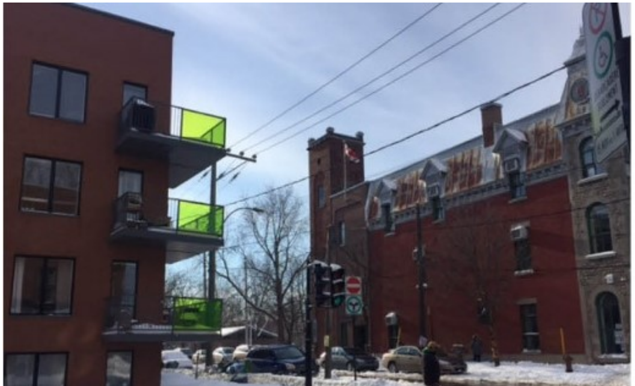
Figure 13. Image showing clear contrast and clash between the different colors and characters of the buildings (Source: the author, Mtl, Qc, October, 2018)
