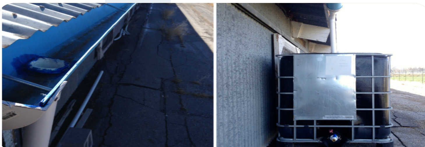
Top view of 6-inch PVC pipe gutter system attached to shed roof catchment area & side view of water storage container with PVC gutter and downspout.
