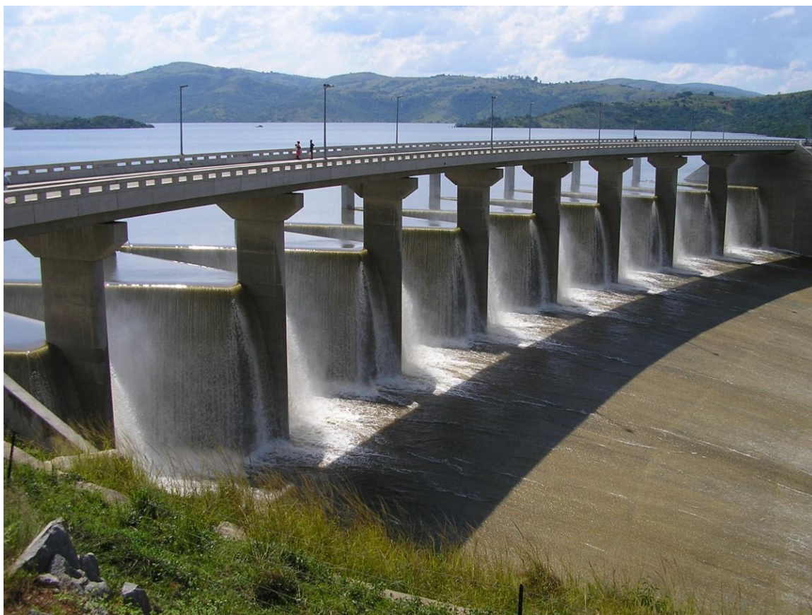
Fig. 2 Maguga Dam arced labyrinth spillway, Hhohho, Swaziland.
