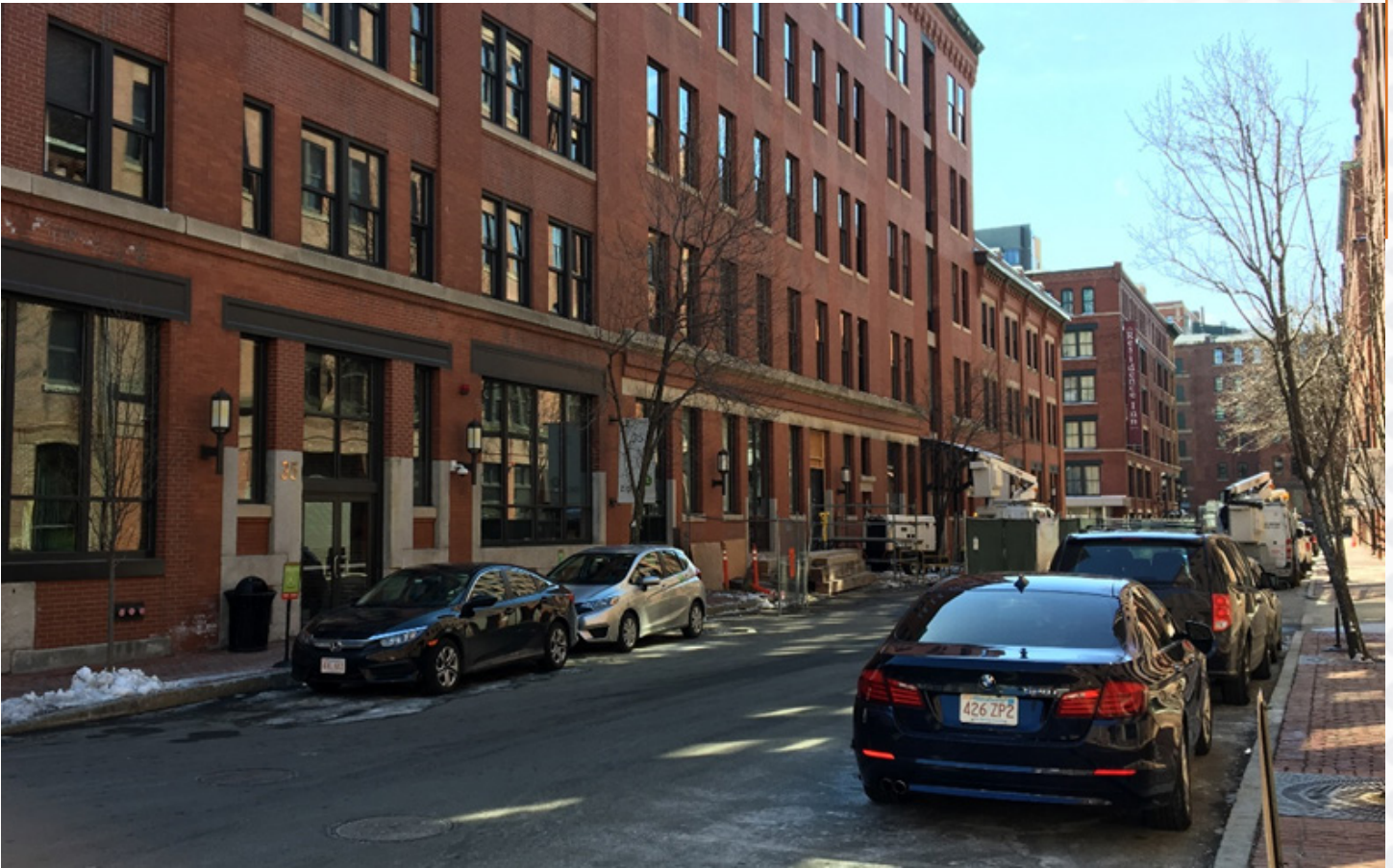
Figure 6-6. Warehouses turned Innovation Space in Fort Point.
