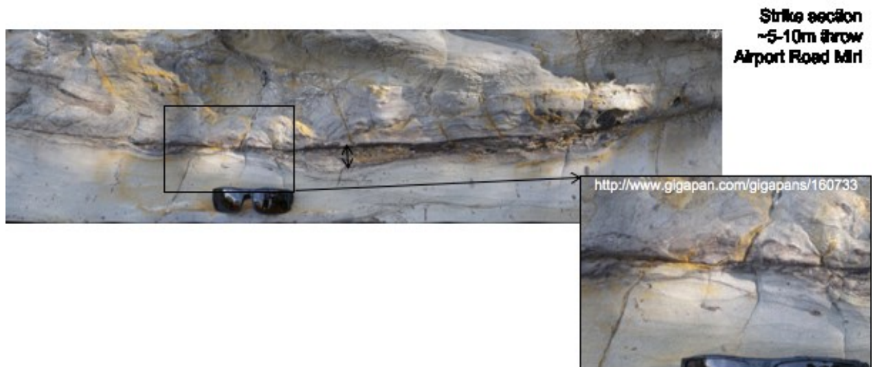
Figure 1 Strike outcrop view of faults at Airport Road Miri, Miri, Sarwak, Malaysia. It shows significant lateral variations in fault rock over the decimetre scale. A high resolution example of this image can be seen at http://www.gigapan.com/gigapans/160733
