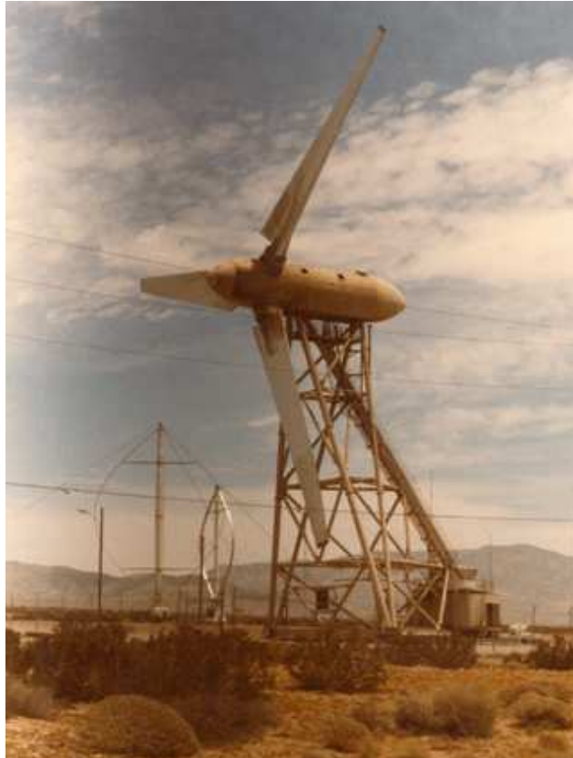
Figure 1.6: Photo of the Bendix SWT-3 experimental wind turbine which was put into operation in 1980s. This figure is taken from [110].
