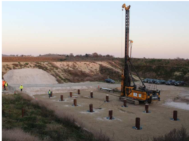
Fig. 5. Driving of FBG instrumented 508mm OD piles at St. Nicholas-at-Wade.
