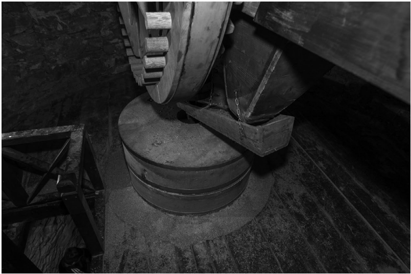
Figure 6.2 The windmill restored, interior, August 2012
