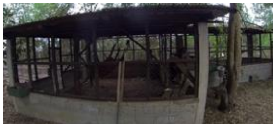
Figure 2.6 Front view far right enclosure
