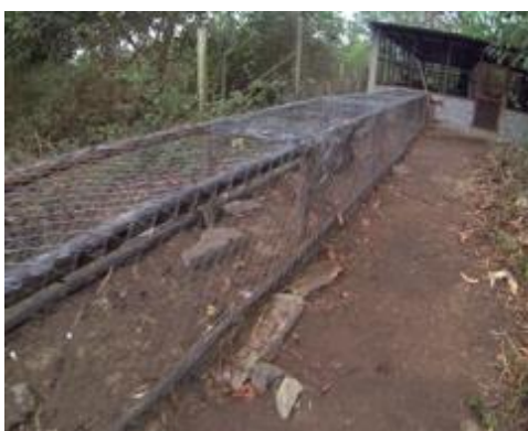
Figure 2.8 The original chain-link corridor linking Enclosures 1 and 3
