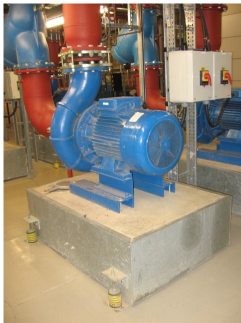
Figure 46 – Water pump plinth and spring supports
