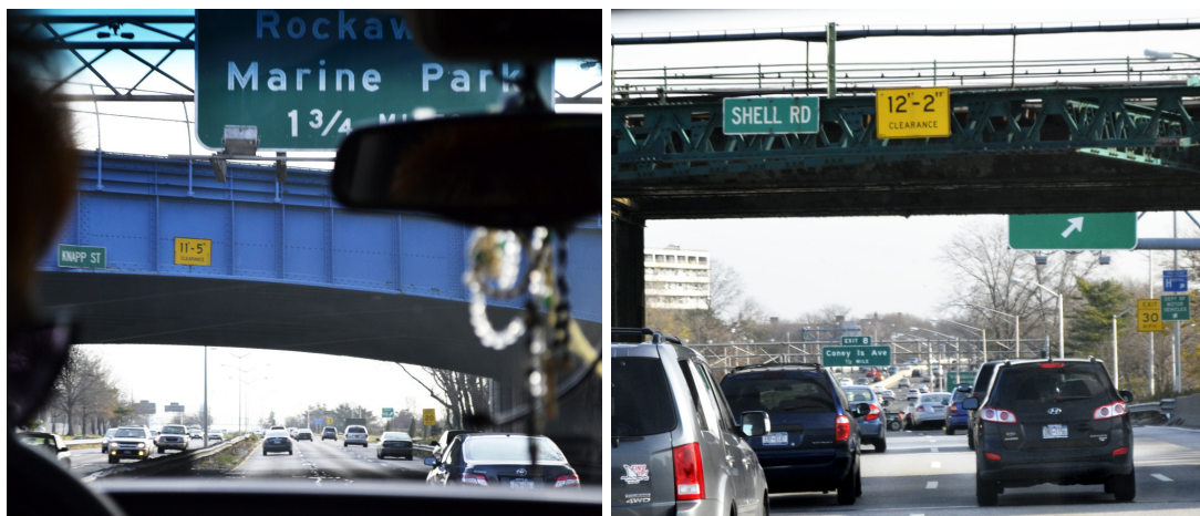
Figure 1: Low bridges over the Shore Parkway, Brooklyn / Queens. Photos by the author.
