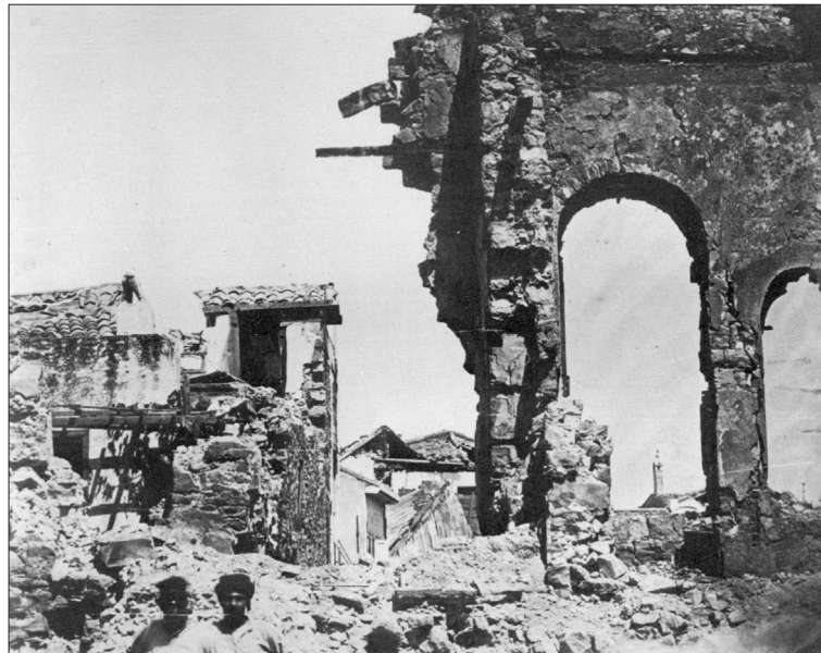
Fig. 6. Chios town: the Aplotaria commercial centre after the 1881 earthquake (Fasoulakis and Bouras, 1983).
