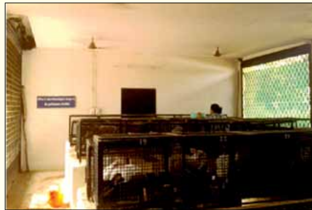
False ceiling made in rabbit shed to reduce heat stress
