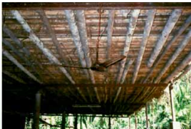
Arrangement of false ceiling in cattle shed in the field
