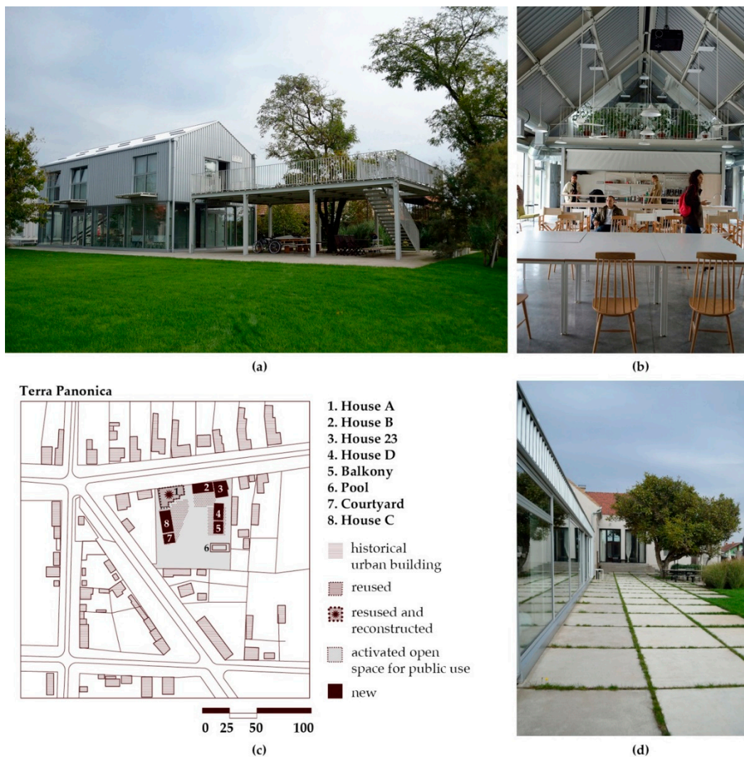
Figure 2. Terra Panonica in Mokrin village—modern cultural and touristic center for creative industry: insertion of new contemporary buildings and preservation of existing traditional houses, (a) Modern design of the house D; (b) House C for indoor events; (c) Spatial layout of the compound; (d) New house C in relation to the reconstructed house A.
