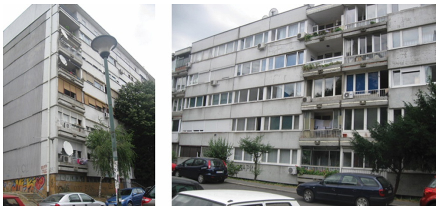
Figure 1. Examples of typical façades of the buildings from the sixties
