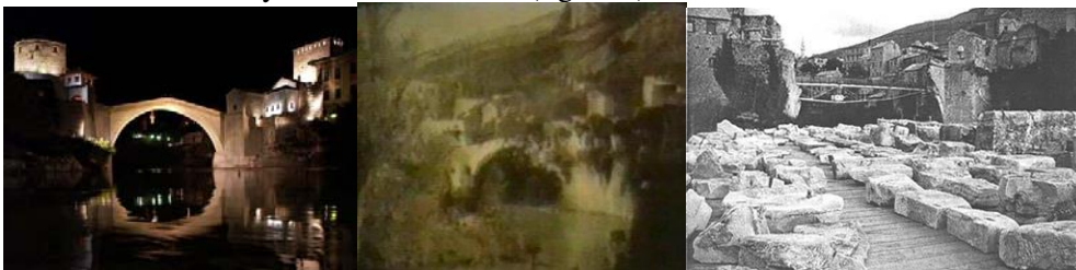
Figure 2. Mostar bridge after the reconstruction, at the moment of destruction, and just before the reconstruction.
