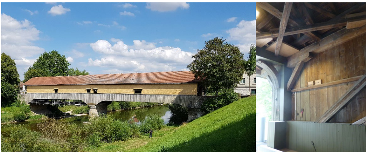
Figure 30: Bridge crossing the Thur in the village of Andelfingen with a view on the instrumentation and two dummy blocks on the north side of the bridge
