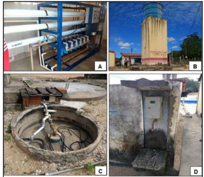
Figure 12 – Equipment related to the stages of the desalination process in the Uruá Community. A) Reverse Osmosis Desinilator; B) Fountain with raw water reservoir; C) Well location; and D) Location point of the freshwater catch.
