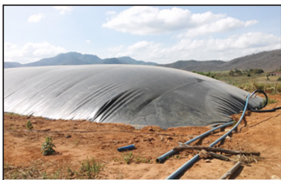
Figure 5 – Canadian biodigester in the municipality of Redenção, Baturité Massif, Ceará
