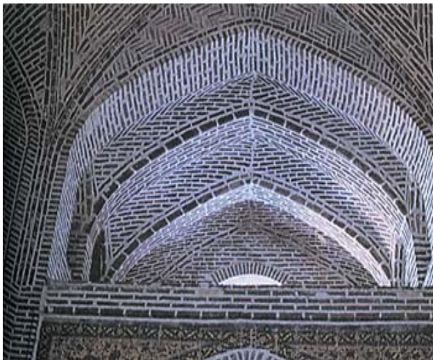
Figure 7: Vault and Toizeh at the north part of the Masjedannabi
