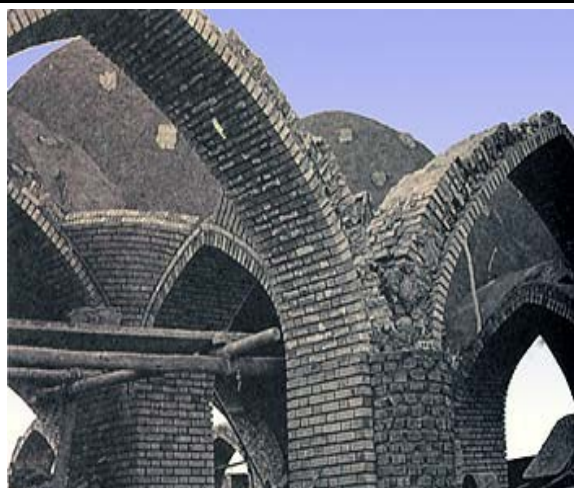
Figure 9: Run the Klonbeh vault in Imam Ali masque in Yazd city
