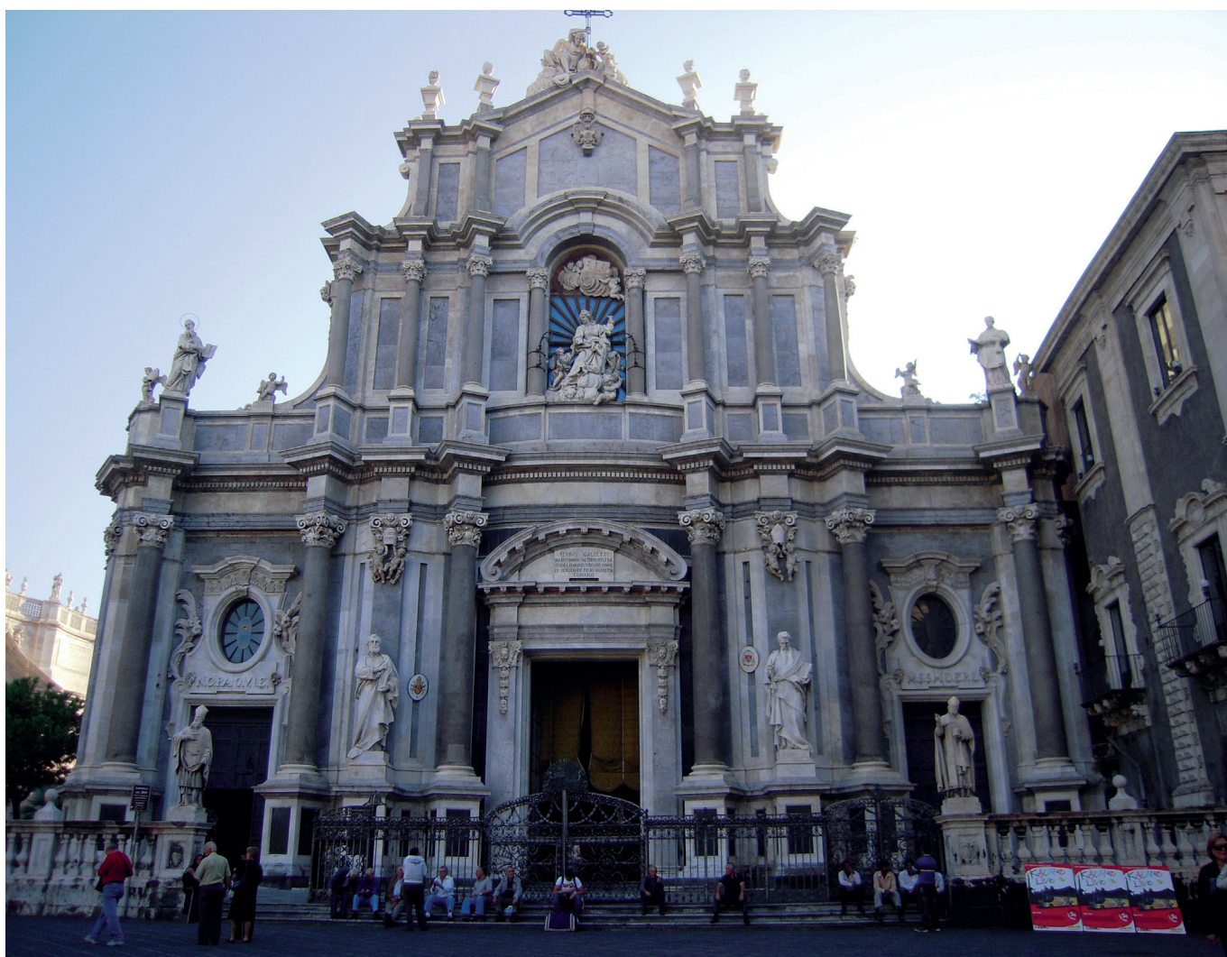
Fig. 5. Catania. Façade of the Cathedral with "pietra di Billiemi" columns and stones on the second order. Author.
