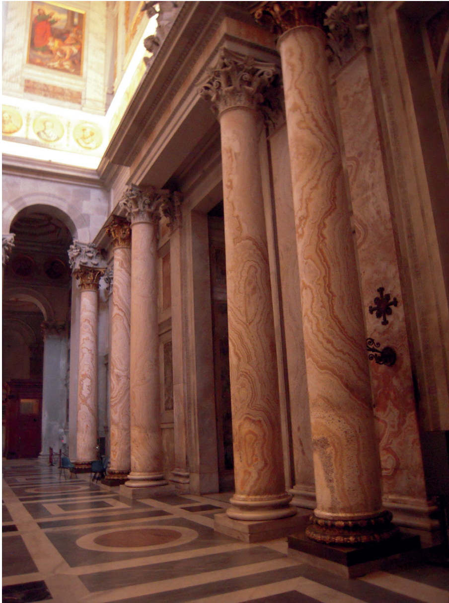
Fig. 1. Rome. San Paolo fuori le mura. Columns on the inside façade wall in "cotognino" alabaster from Egypt. Author.
