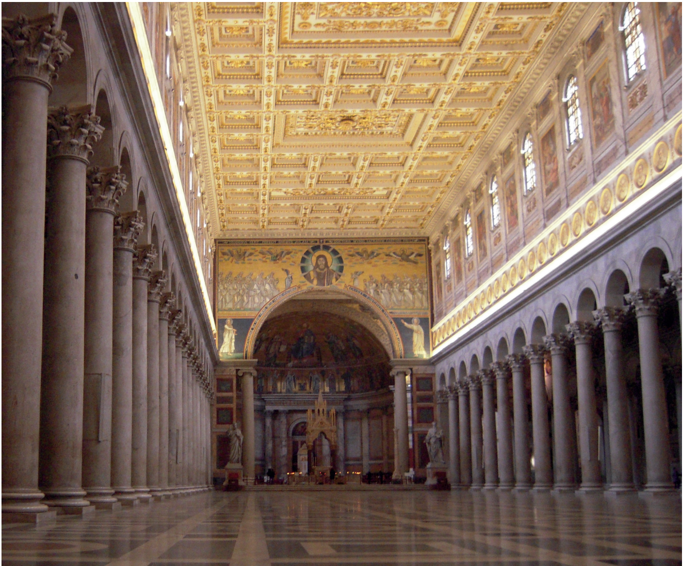
Fig. 2. Rome. San Paolo fuori le mura. Columns of the nave in Montorfano granite and triumphal arch with Baveno granite. Author.
