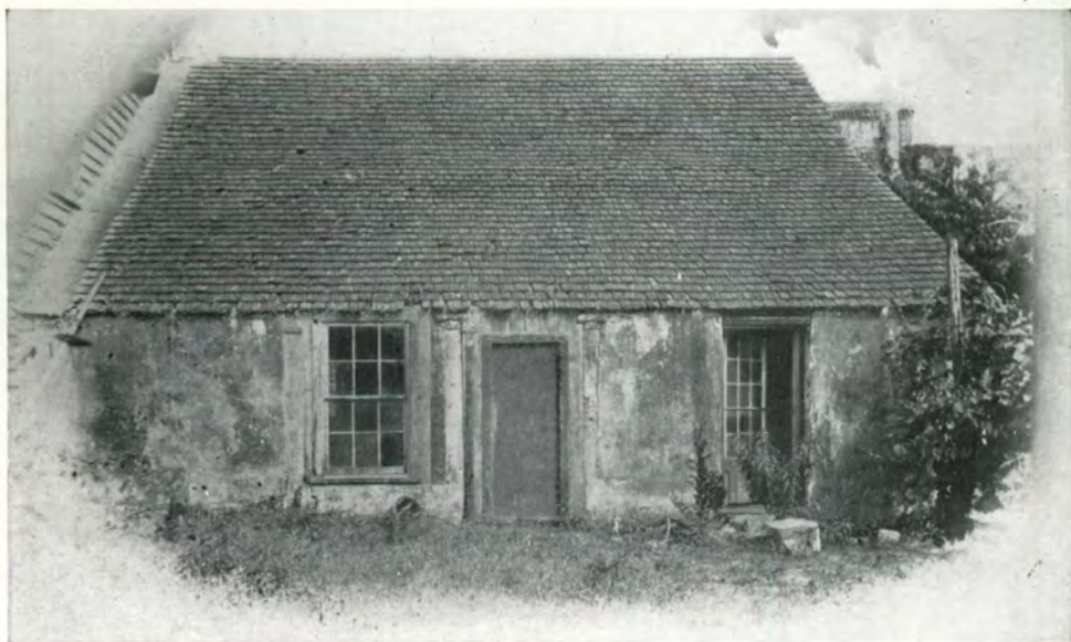
REAR VIEW OF THE OLD HOUSE ON ST. GEORGE STREET.
