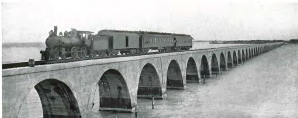
LONG KEY VIADUCT. ON THE EXTENSION. 10,444.65 FEET BETWEEN ABUTMENTS.
