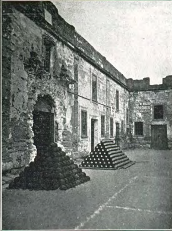
CHAPEL ENTRANCE AND CASEMATES.
