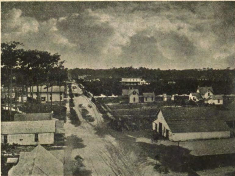
THE NORTH BOULEVARD AND WEST NEW YORK AVENUE IN THE EIGHTIES
