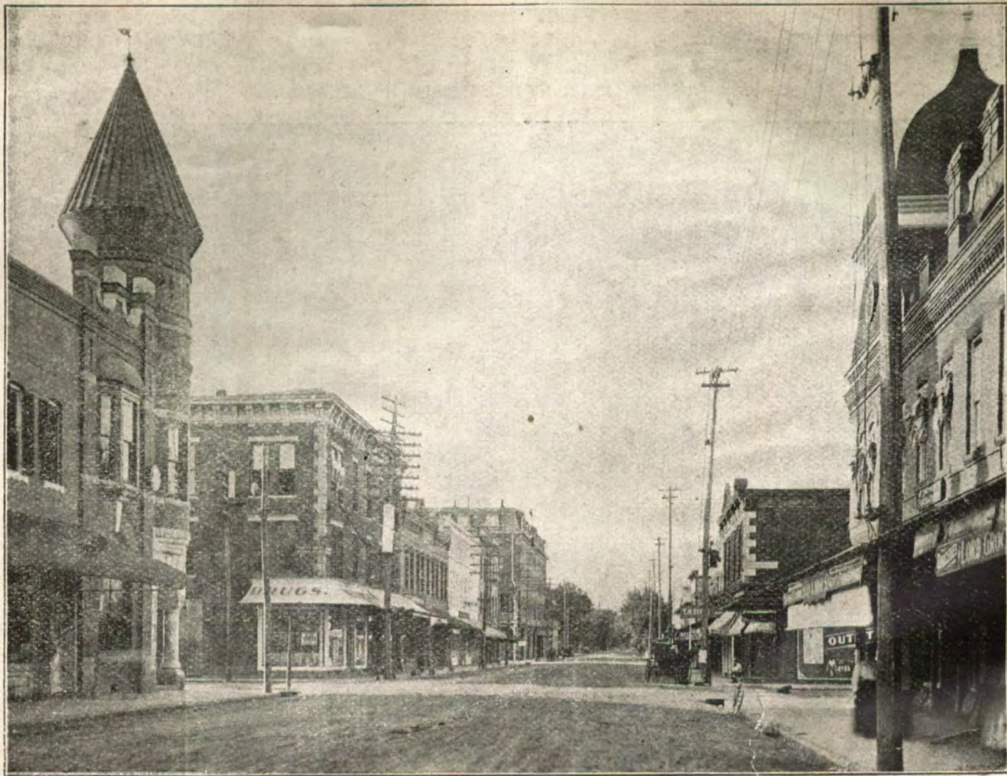
ORANGE AVENUE, LOOKING NORTH
