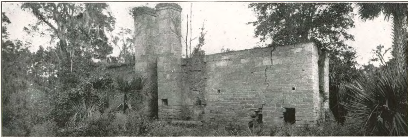
Ruins on Tomoka River, believed to be the Mission of San Antonia de Anacape, built in 1655. The arches of coquina rock were closed when the building was used as a sugar mill during the English occupation.
