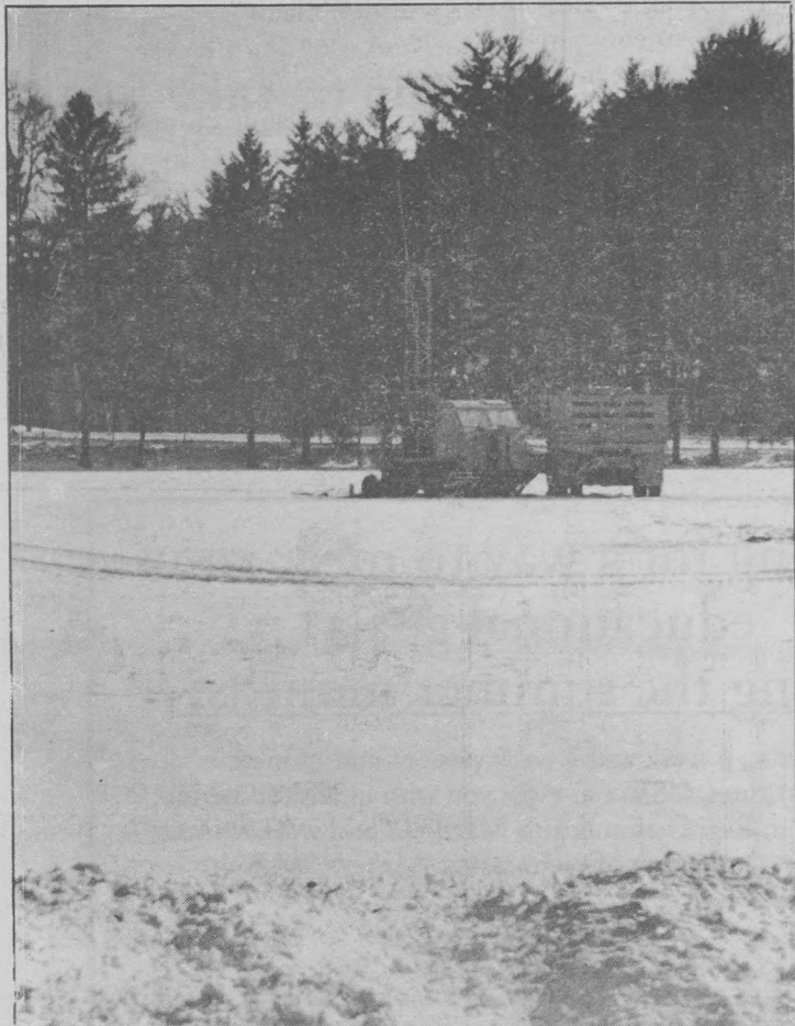
Plans for building the new dormitory are underway as evidenced by equipment on the field. Alexis Gentile photo.
