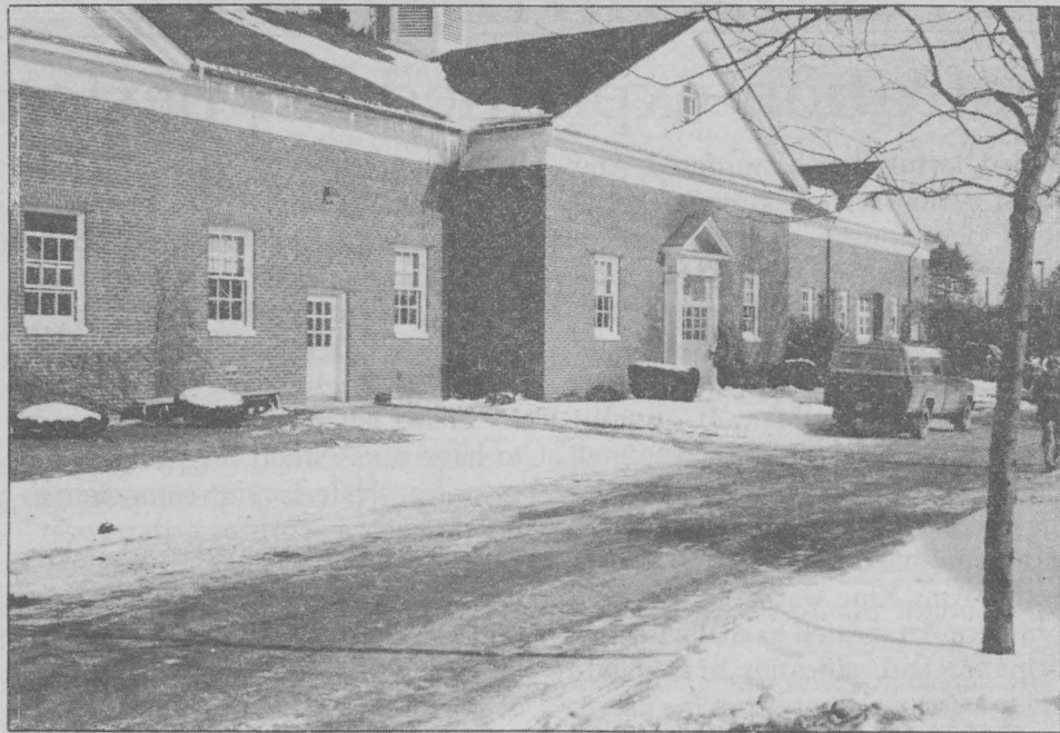
Due to its central location, the Maintenance Center is expected to be replaced by a student center. Alexis Gentile photo.
