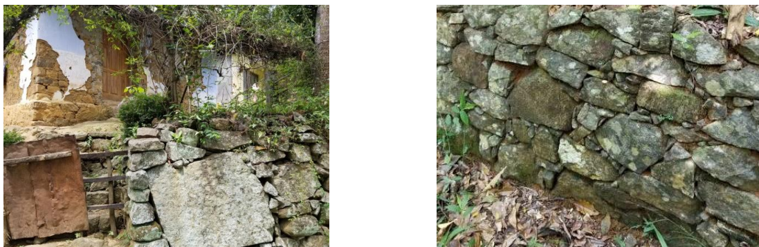
Fig. 7. Retaining Walls. Source: Author.
