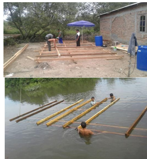
Figure 1. Installation of floating net frames
