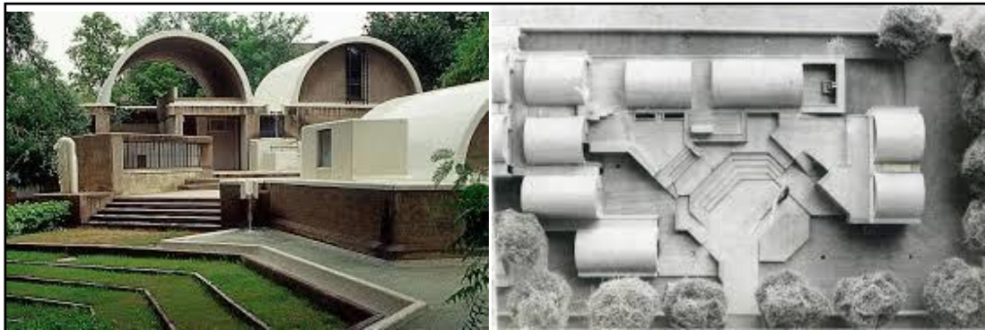
Figure 2. The roof of the local mosaic at Sangath Doshi.
