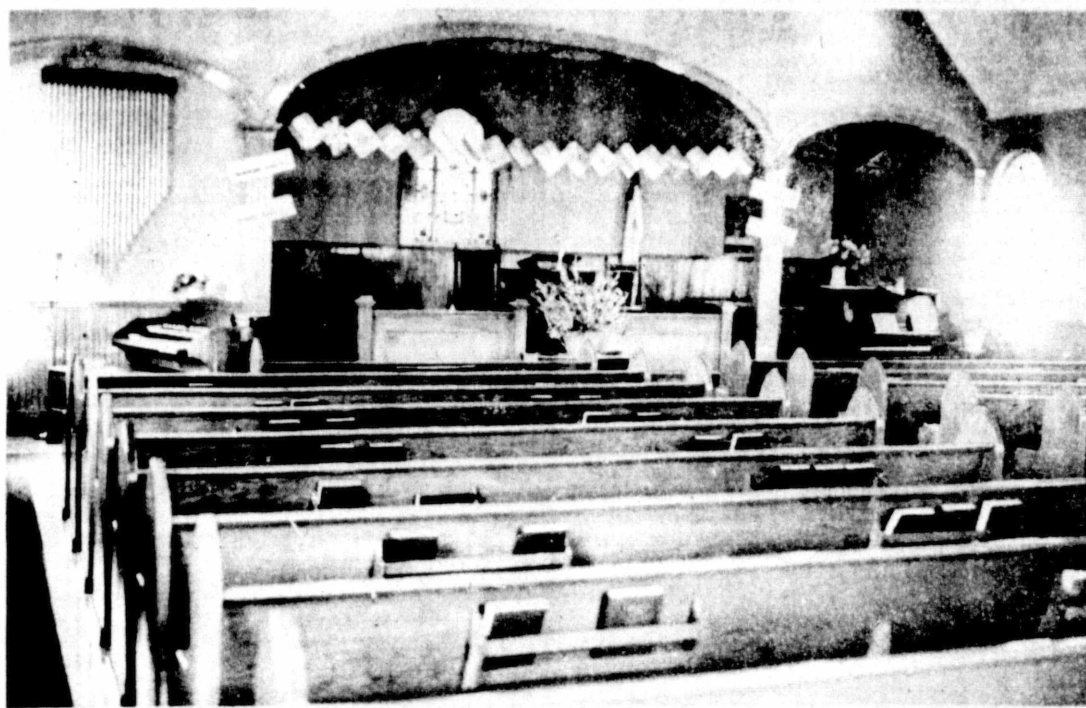
CHURCH IS RENOVATED—Work on renovating the Christian and Missionary Alliance Church at Pleasant street and Highland avenue is continuing, although work on the main part of the church has been completed. The sanctuary, shown above, has been completely repainted and varnished. At the time of the photo this week, the church was decorated for the Missionary Convention that will begin Sunday. Outside work has included a new entry, new steps will be installed, and the building will either be painted or given new siding. (Pioneer Times Photo)
